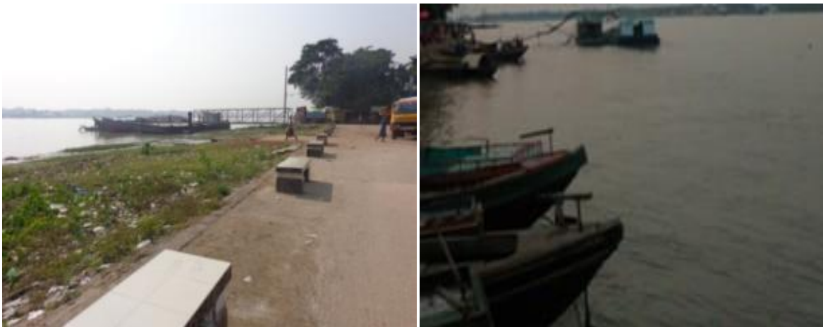
Existing Pontoon for CSD
