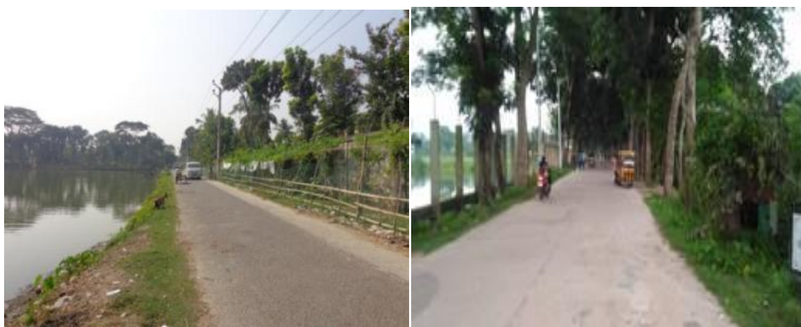
Road by the side of Barishal CSD and proposed site
