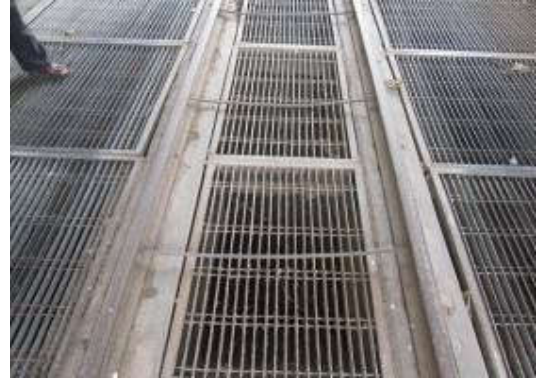
(b) Receiving point of dropping wheat grains after opening the bags of wheat (in operation at present)
