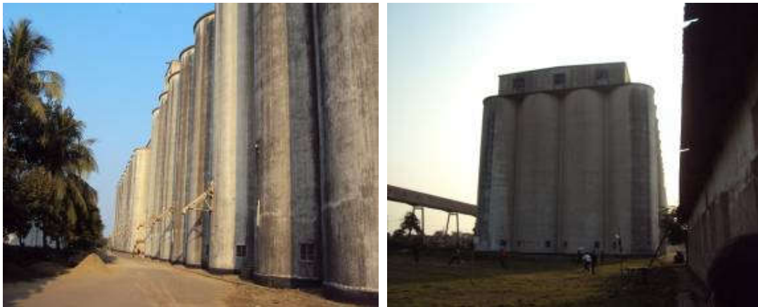
Figure 7-13 Chittagong – Concrete Silo
