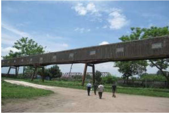
(a) Conveyer gallery to receive food grains from river vessels (presently not in operation)
